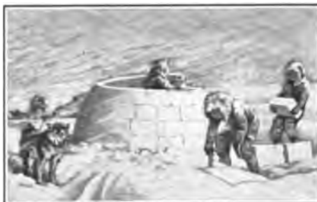
"It is made of snow blocks piled up in a ring"
